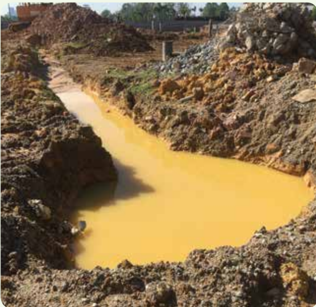
Temporary sediment pond at W City JGCC project site to capture eroded or disturbed soil from entering watercourse.
