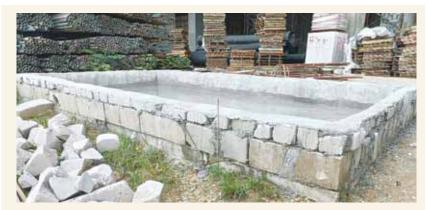
Surplus bricks are reused as bunds to prevent oil spillage from the IBC tank
